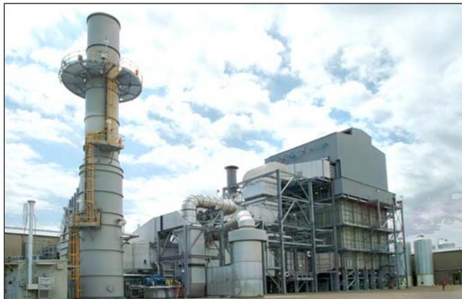
*Hydrogen plant in Edmonton, Alberta is the most modern hydrogen plant design to date with a capacity in excess of 168 tpd (70 MMSCFD) of hydrogen with steam export.*
