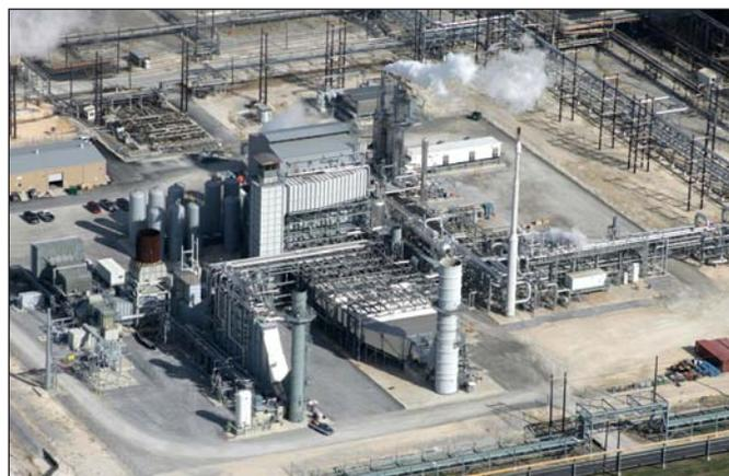
*Excellent hydrogen supply reliability can be maintained from facilities such as Air Products' Port Arthur, Texas complex with **two SMR hydrogen plants** producing 105 and 110 MMSCFD of hydrogen respectively, totaling 516 T/D or 239,000 Nm<sup>3</sup>/h of hydrogen, each with integrated power generation.*
