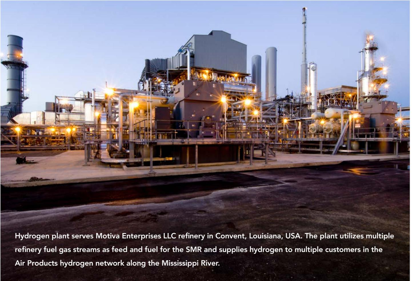
Hydrogen plant serves Motiva Enterprises LLC refinery in Convent, Louisiana, USA. The plant utilizes multiple refinery fuel gas streams as feed and fuel for the SMR and supplies hydrogen to multiple customers in the Air Products hydrogen network along the Mississippi River.
