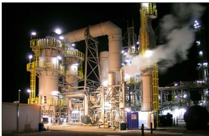
*Hydrogen plant near Cressier, Switzerland services Petroplus refinery, with a hydrogen capacity of 7.1 MMSCFD (17 T/D ; 7,850 Nm<sup>3</sup>/h) on butane feed.*
