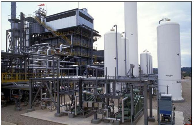
This plant in Tarragona, Spain incorporates a pre-reformer to process naphtha or refinery fuel gas for the Repsol refinery. In addition, Air Products recovers CO<sub>2</sub> for the merchant gases market in Spain.
